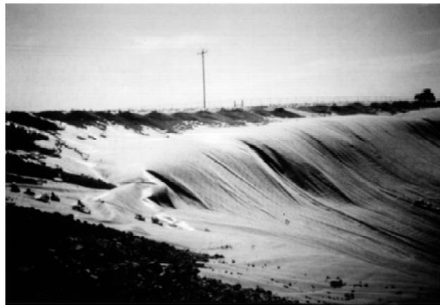
Figure 1. Examples of geomembrane uplift.
