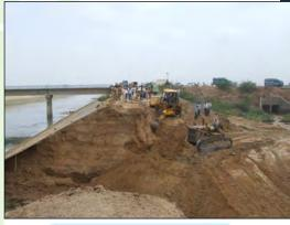
Embankment Section - Stratified Strata without Zones and Filters
