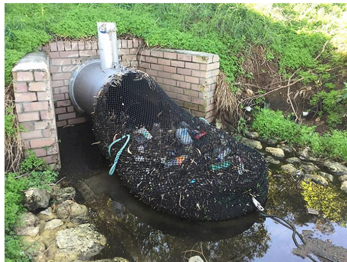
A net safely captures waste plastic from a drain
