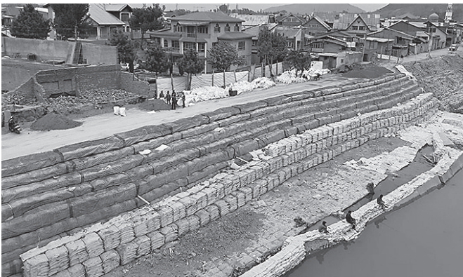
Fig. 5 - River erosion protection using geosynthetics under construction.
