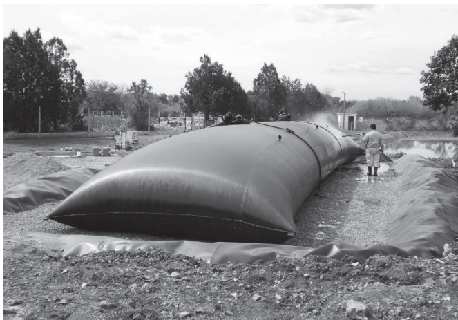
Fig. 8 - Geotextile tubes used capturing and further dewatering sludge for disposal in solid form.
