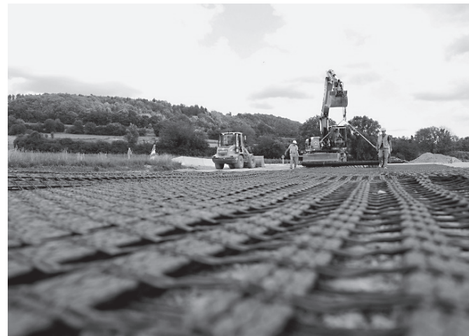
Fig. 4 - Geosynthetics reduce aggregates use in road building.
