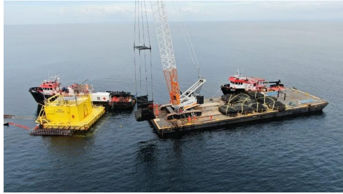
Figure 4 – Geobag Lifting Harness and Installation
