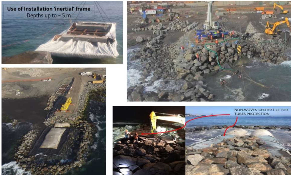
Figure 3. Construction detailed sequence
