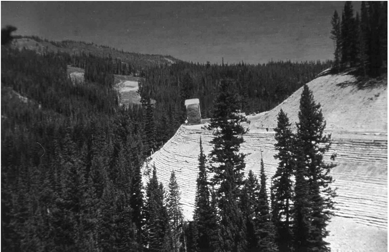
Construction of a geosynthetic-reinforced steep slope to widen roadway through Idaho National Forest
