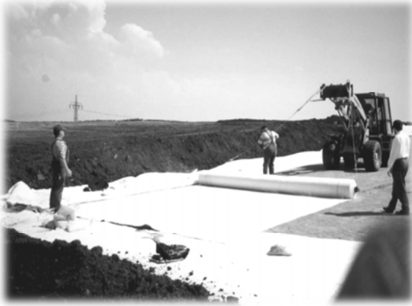
Installation of a GCL in the cover of an MSW landfill
