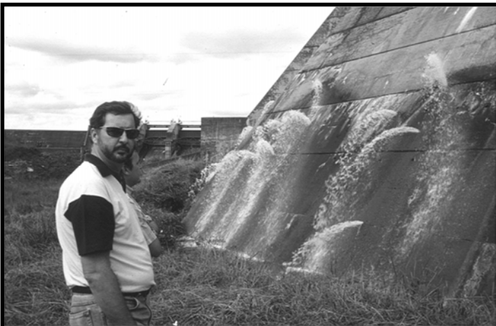
Concrete dam leaking!
