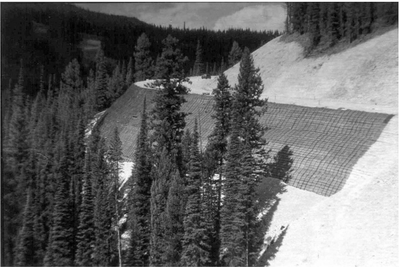
Erosion control mat placed to promote vegetation and protect the exposed facing of a geosynthetic-reinforced steep slope
