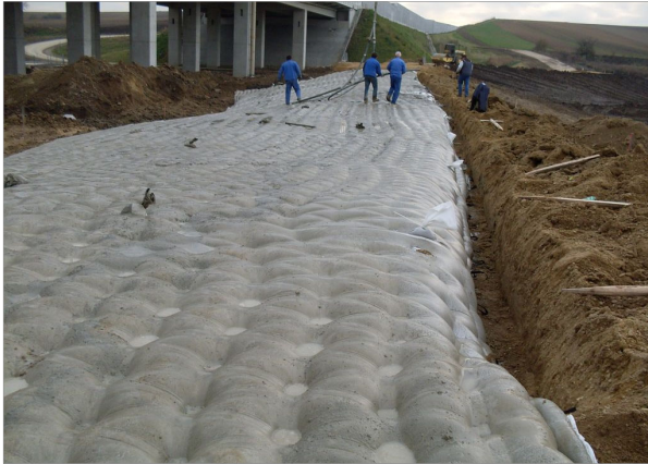
Crest with anchor trench (concrete slab)
