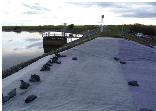
Levelled crest (covered with nonwoven)
