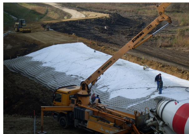
Filling of the mattress (stepwise)
