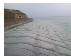
3. Filling of the mattress with highly fluid concrete/mortar
