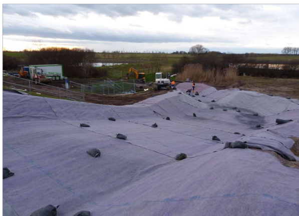
Levelled channel (covered with nonwoven)
