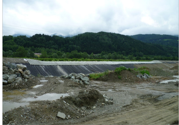
After completion (air side)
