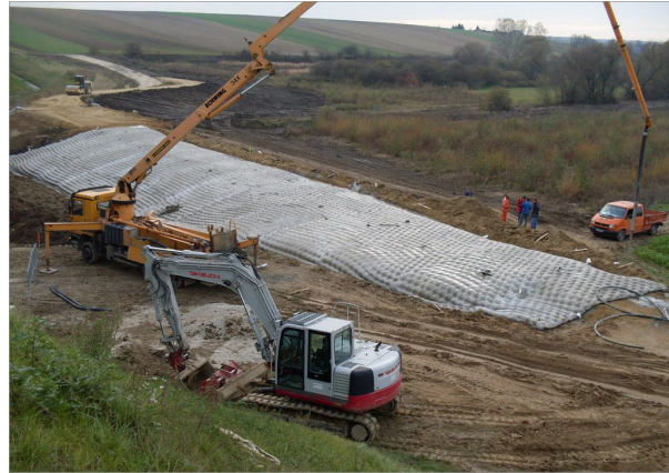
After filling (duration 7h with 5 workers)
