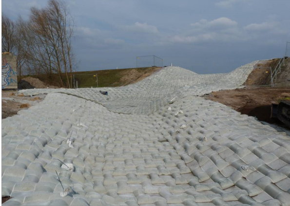
Channel after installation of concrete mattress
