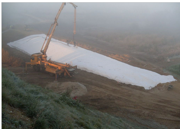
Empty concrete mattress (lay-out in 1h with 5 workers)
