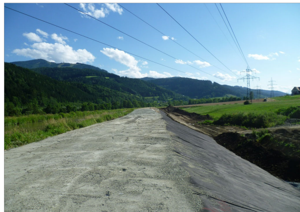
Levelled subsoil
