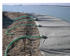
2. Lay out of the pre-fabricated panels
