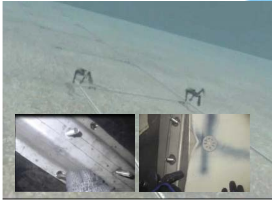
Installation of anchoring stainless steel profiles
