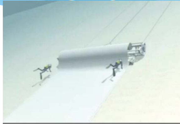
Installation of geogrid, geotextile, PVC geocomposite
