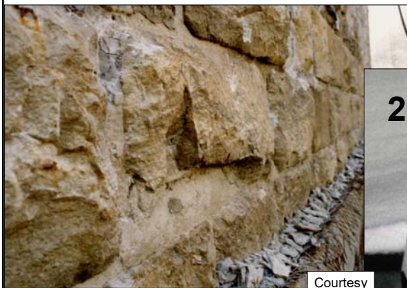
Camposecco Dam, Italy
