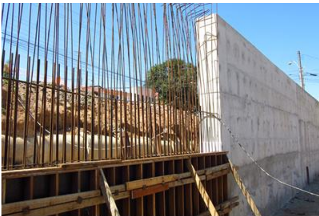
Reinforced Concrete Wall
