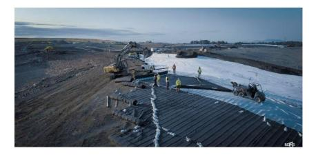
These barriers, drains and other geosynthetic materials are designed to perform robustly for centuries. Over the past 60 years, they have successfully contained waste, protected groundwater and provided sanitation.
