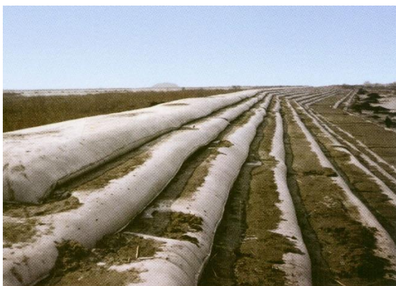
e. Geotextile tubes as slope revetment [PIANC 2011]
