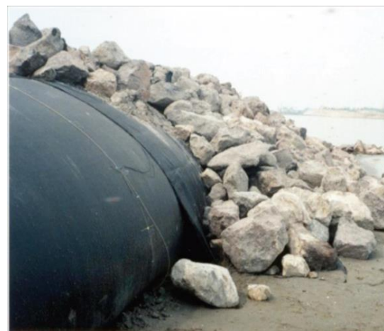
f. Covering of a Geotube [TenCate USA]
