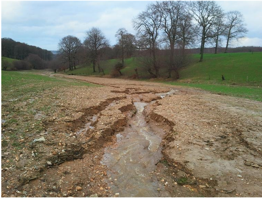
Figure 1. Erosion with gully formation [Province of Limburg, Belgium]
