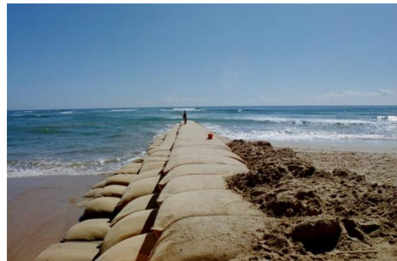
d. Groin, core made of geosynthetic bags. Maroochy, Queensland, Australia [Restall et al., 2002]
