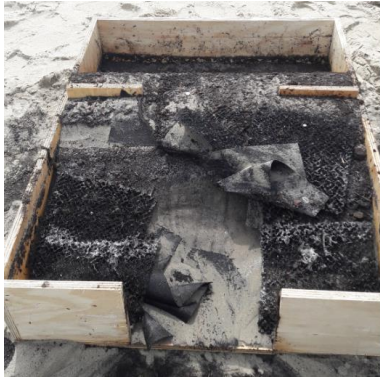
c. Sheetting and geogrid
