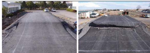
**Fig. 2:** The results of road structures due to settlement, with (a) CRE method, (b) traditional method (Ohta et al., 2013)
