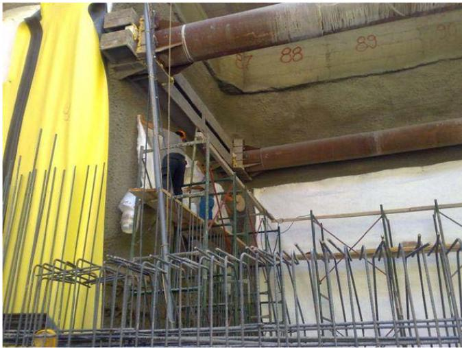
Figure 3: Cushion geotextile installation
