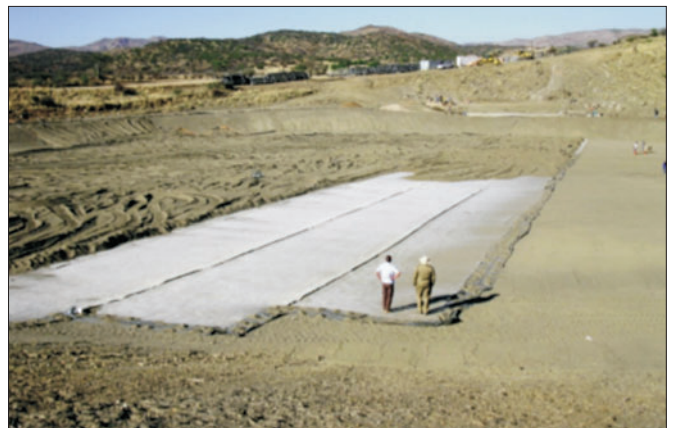
The new GCL-lined cell at Kupferberg under construction
