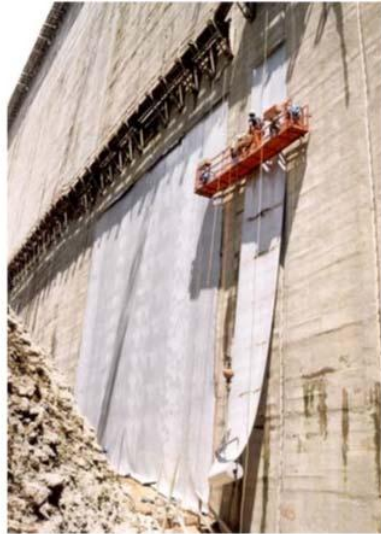
Lining the upstream face of a dam (*)
