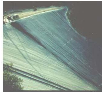
Geomembrane-lined dam (*)
