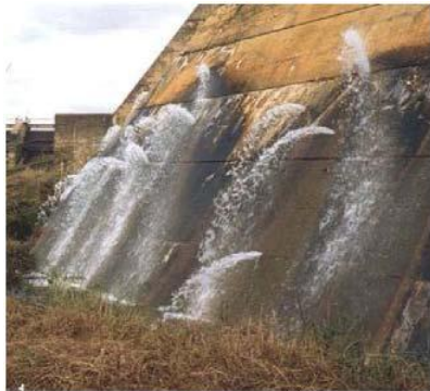
Leaking dam (*)
