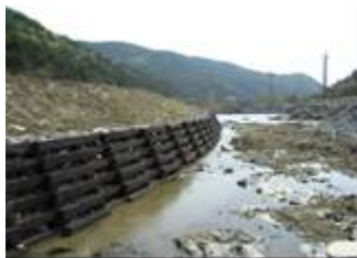
Construction d'éléments PE
