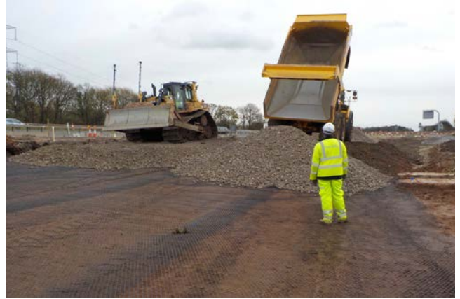
TriAx delivered a bearing capacity at the top of the granular layer of between 60 and 70MPa, higher than the 50MPa required.
