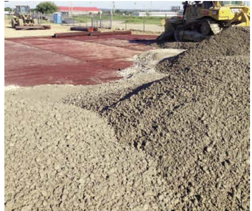
Bridging soft soils and building the platform
