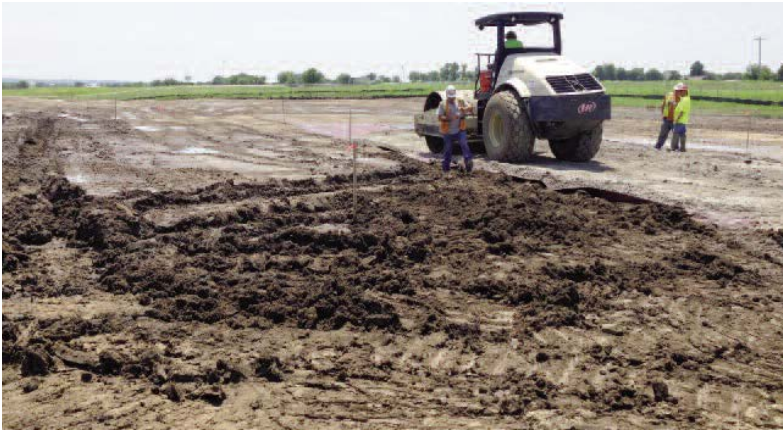
Working the subgrade before placement of Mirafi®RS580i geosynthetic
