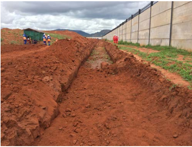
excavating the channel
