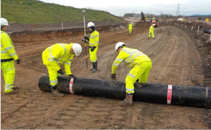
Tensor's TriAx geogrid was used to stiffen the unbound capping layer, as an alternative to lime stabilisation and 'dig and replace' solutions.
