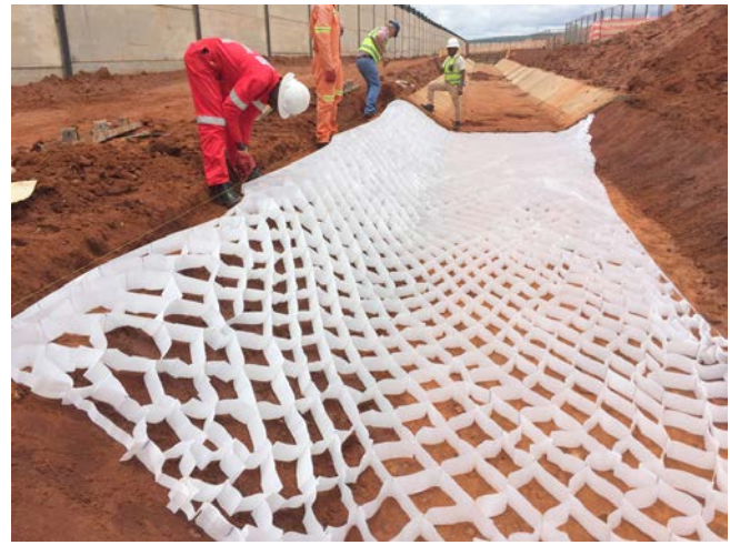
using the the tension frame to peg the Multi-Cell in position
