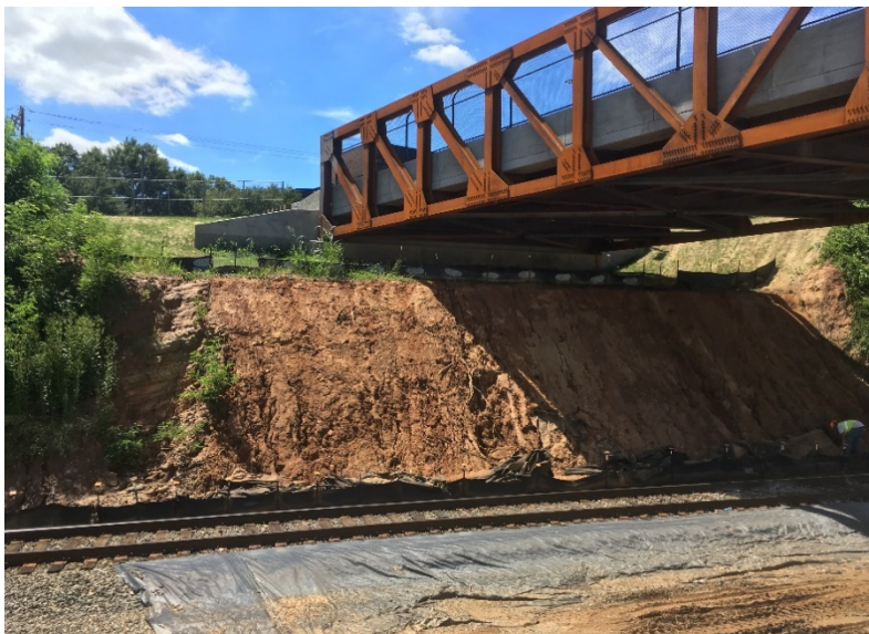
The slope before anchor installation
