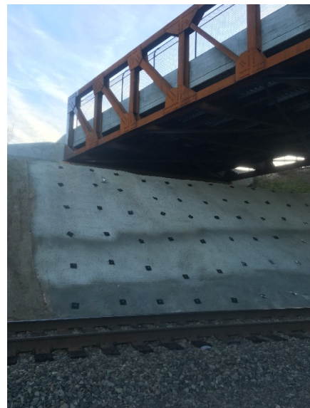
After reinforcement using Platipus Anchors
