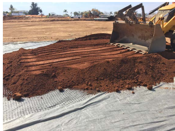
bidim separates the stabilising TriAx from the in situ and the geotextiles were overlaid with 600mm topsoil
