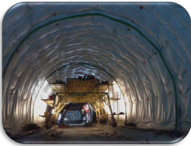
Figure 1 Klokova Tunnel under construction
