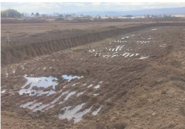
The waterlogged soil was not conducive to heavy plant
