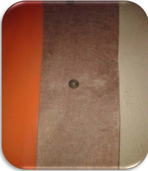
Figure 2a Tunnel lining by a non-woven drainage geotextile
