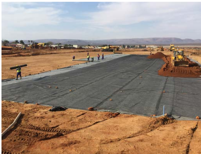
The entire base of the site was stabilised for plant and construction using TriAx and bidim
