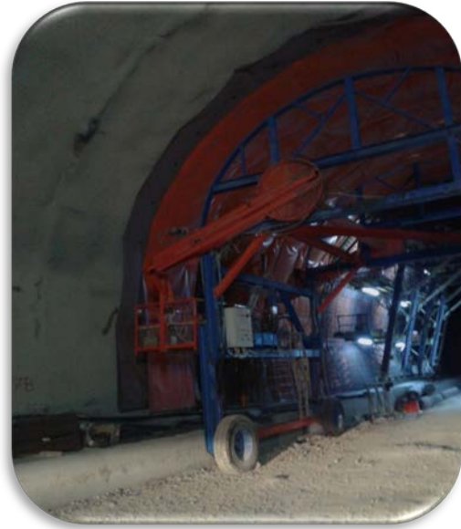
Figure 2b Coverage by waterproofing geomembrane
