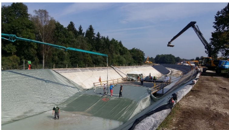
Figure 1: Filling of canal bottom by patented installation procedure
