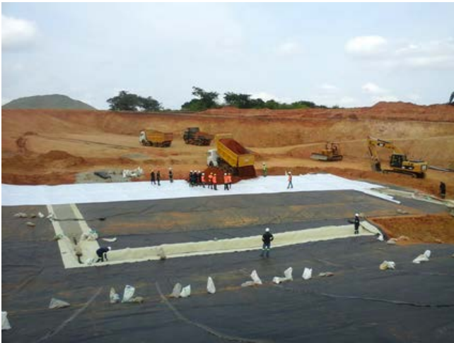
Placement of aggregate leachate collection system over the double-lined geosynthetic base liner system
