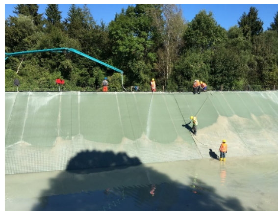
Figure 2: Filling of side slopes, after the bottom section has been filled
