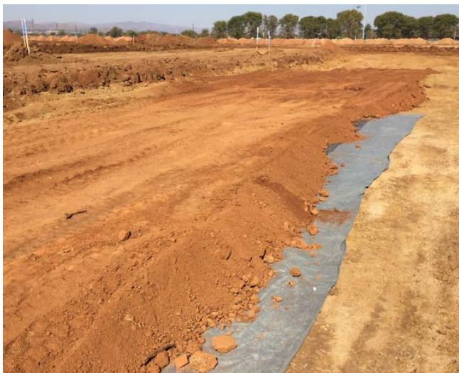
The successfully stabilised trial section
