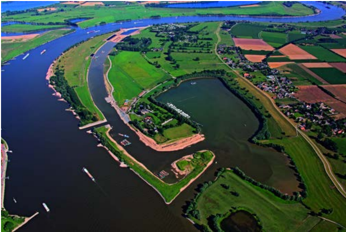
Aerial view of the flood channel
