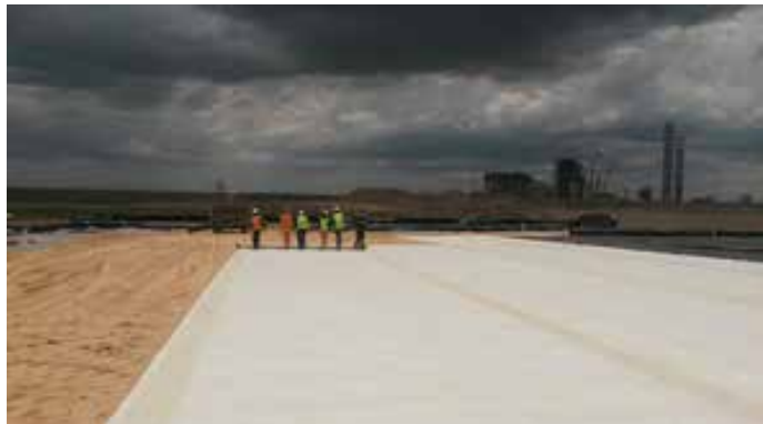
EnviroFix X1000 GCL will contain any potential leakage through the upper layers
