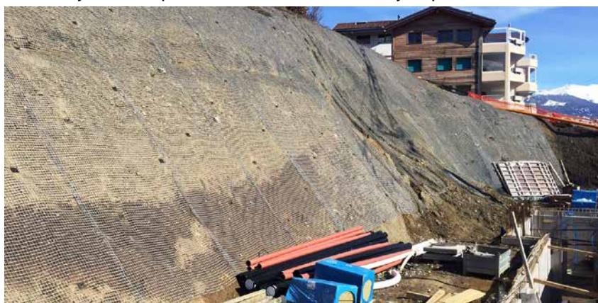
Failure of the slope after construction had started
