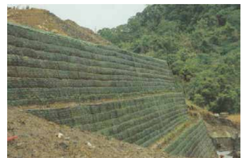
RSS after construction with Green fascia
