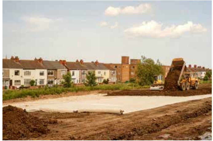
Soil placement on top of GCL
