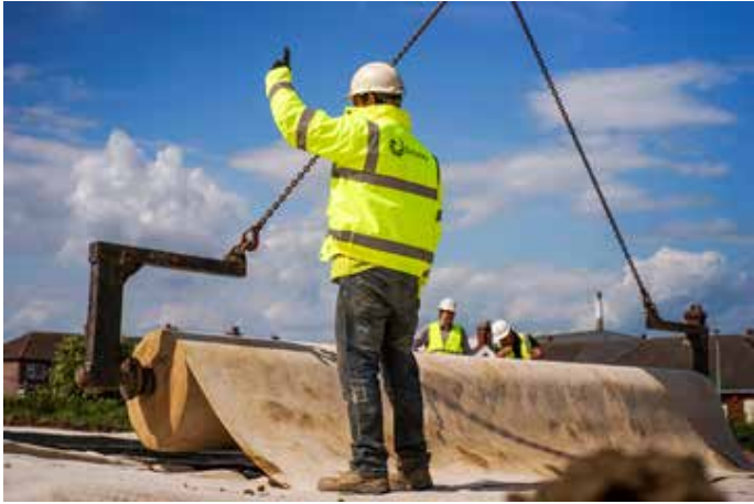
Unrolling and Overlapping of Bentofix® X2 NSP 4900 – a GCL with an additional polymeric coating barrier
