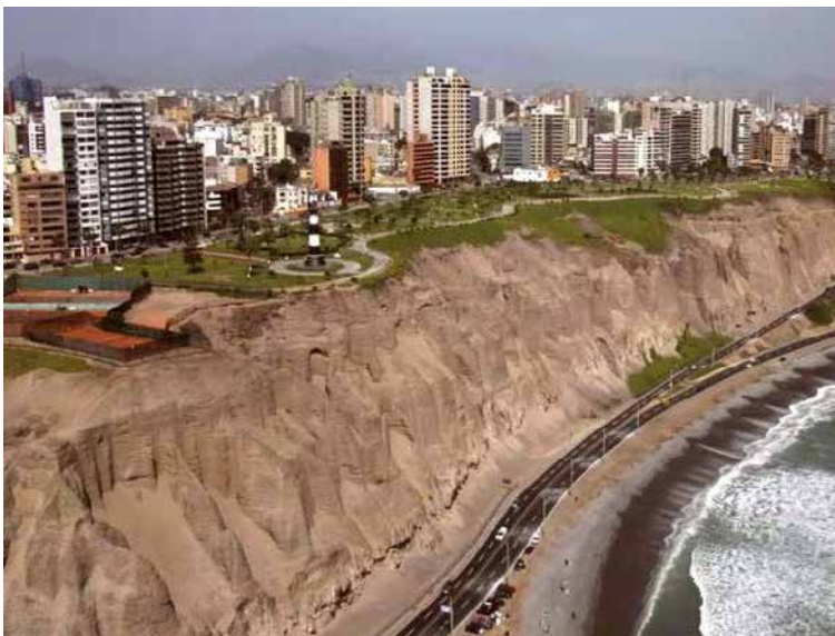
Costa Verde Slopes without protection, a potential danger along an important road.
