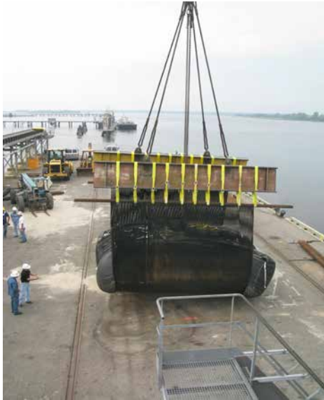
50 m 3 Geobag® Unit Lifting Test
