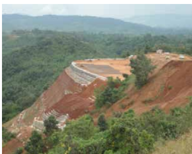
Installation of TechGrid Geogrid
