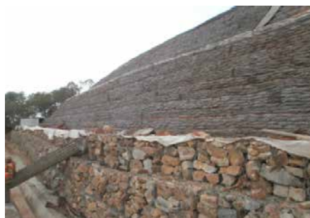
Gabion toe wall
