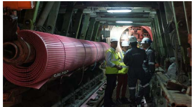
Visit of the STEP sewer tunnel project with CPL being installed
