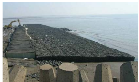
Apron using PP rope gabions
