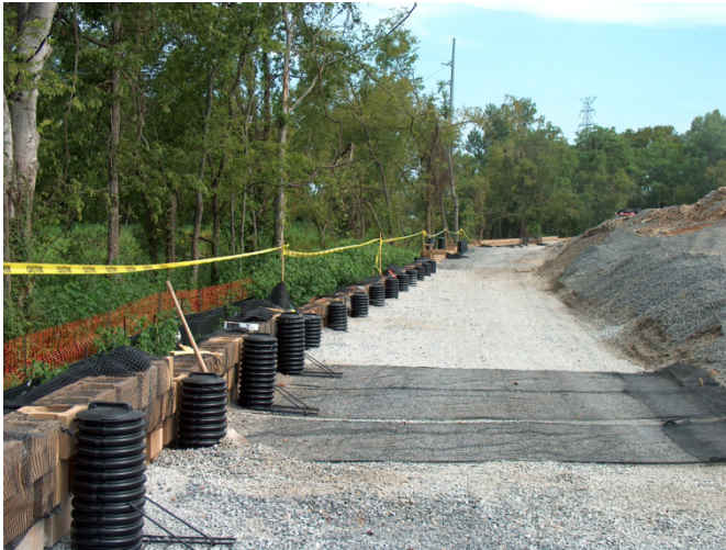
At the top of the wall, 282 Sleeve-it rail integration units were used to stabilize the fence.
