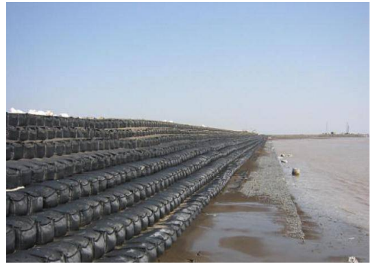
Shore protection work after construction
