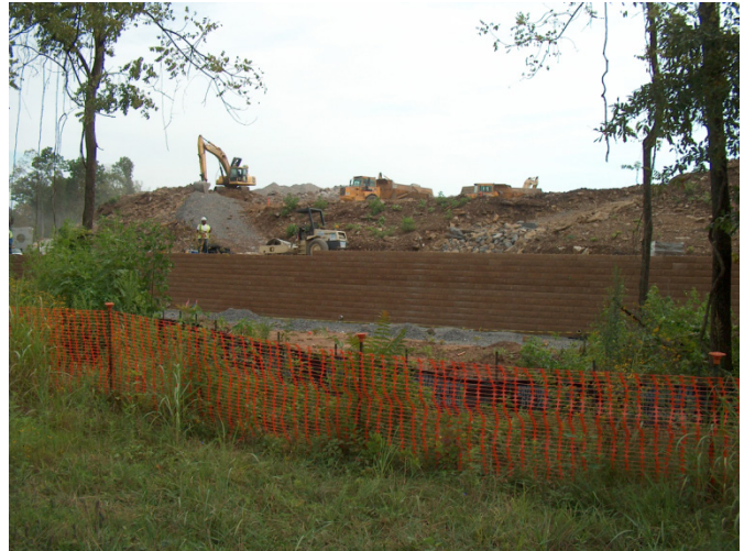
250,000 cubic yards of limestone was removed and 57 cut stone was put in its place for reinforcement behind the wall.
