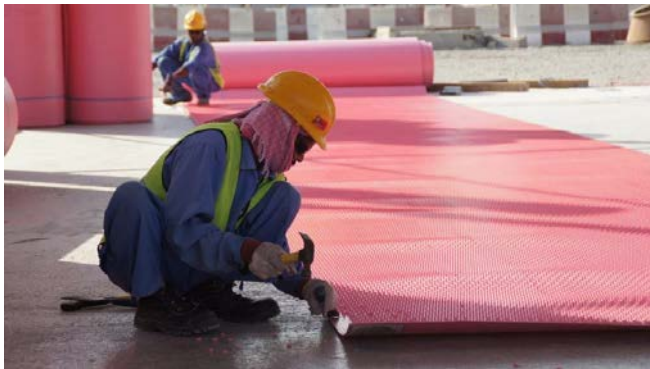
Preparation of concrete protection liner for double wedge fusion welds
