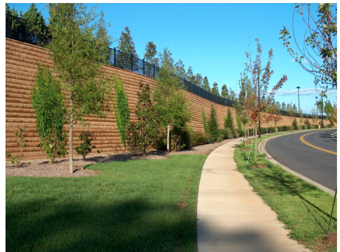
This massive retaining wall with reinforced railings at the new Hendersonville, TN Sam's Club allows for maximum land use while keeping pedestrians safe.
