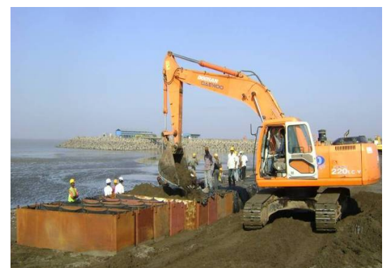
Steel frames to support geotextile containers
