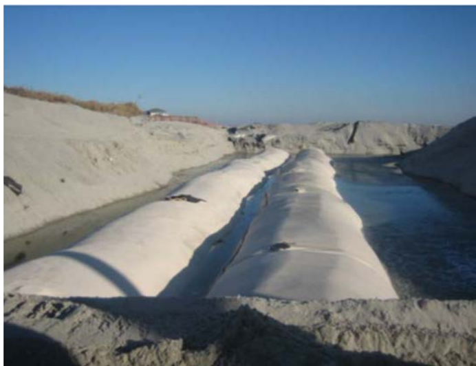
Two parallel Geotube units comprise the bottom layer of the structure. Upon completion of filling the top Geotube unit, sand was placed over the structure and sea grass was planted
