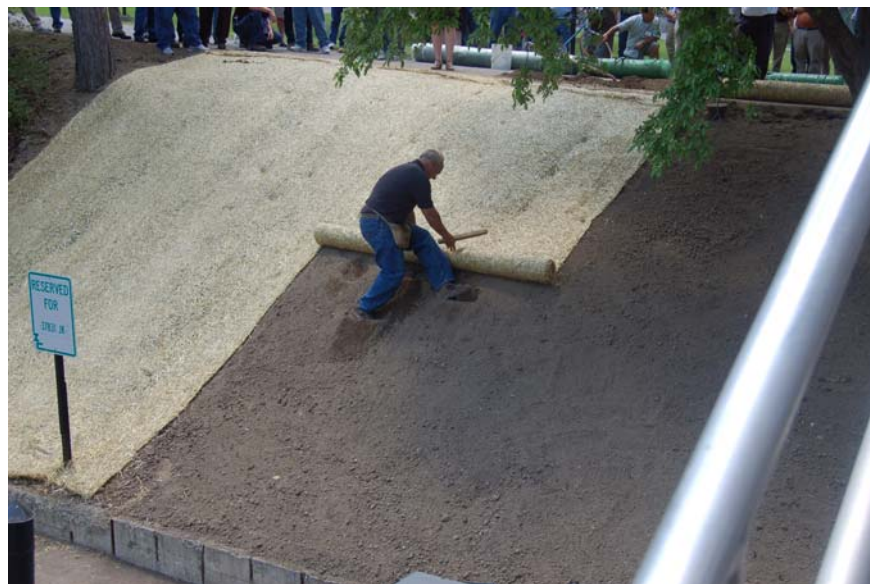
Fig 4 – RECEP Being Installed
