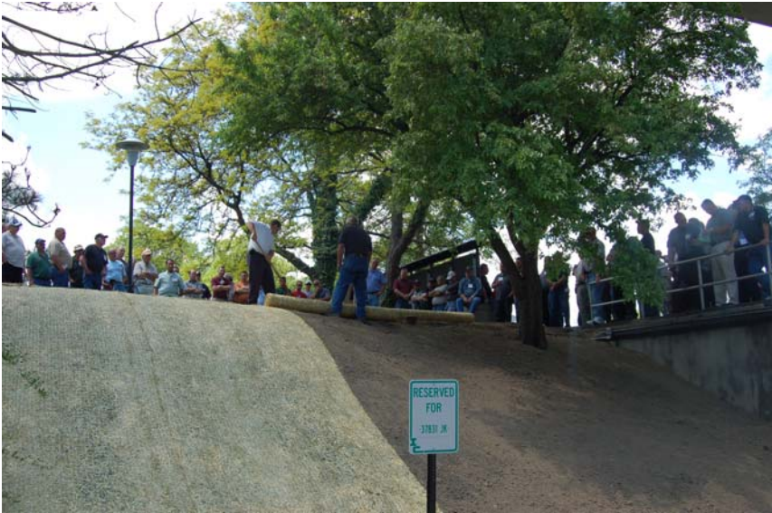
Fig. 6 – Attendees Watching the Installation
