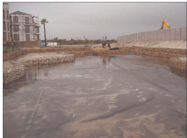
Floor lining being installed after all construction activities completed on site
