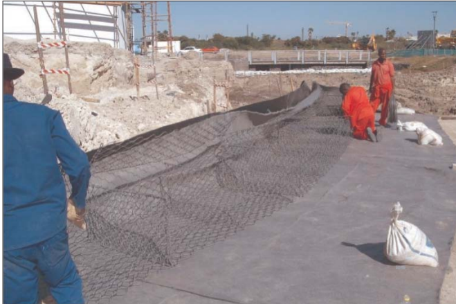
Liner, Bidim and gabion baskets in place around perimeter
