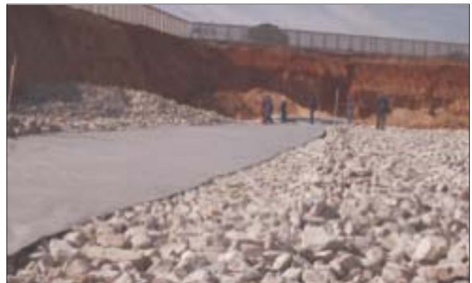
Layer of Fibertex F-50 above dump rock
