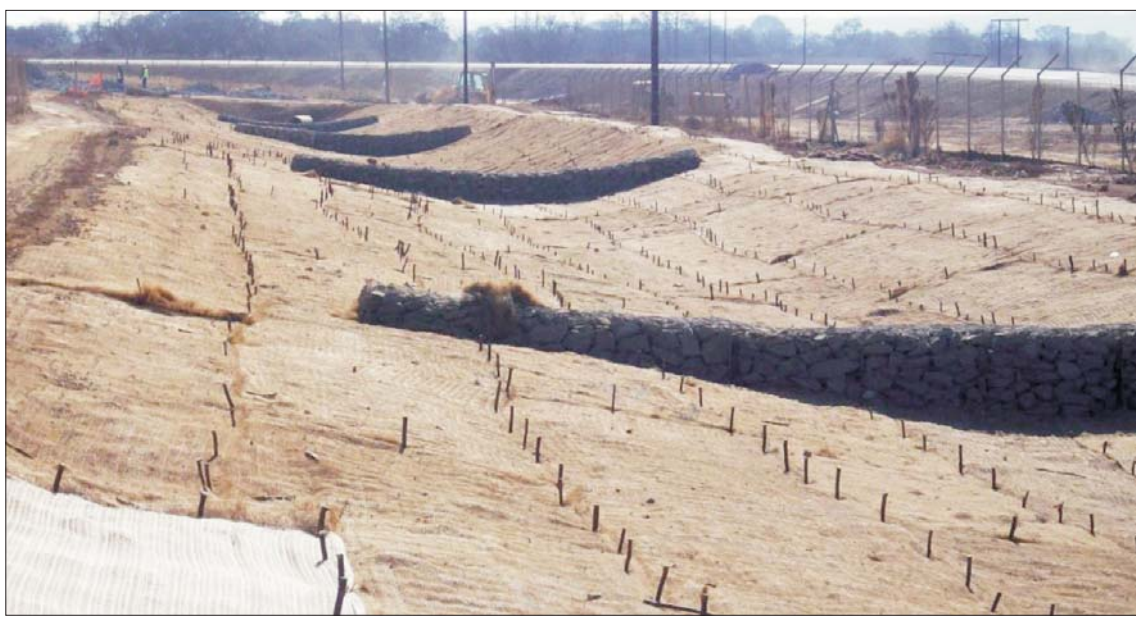
Some of the ECC-2 product being installed
