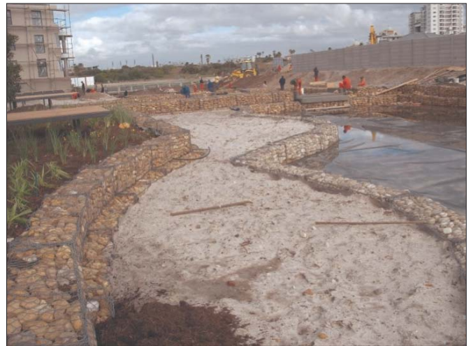
Clean fill and topsoil in place behind gabions
