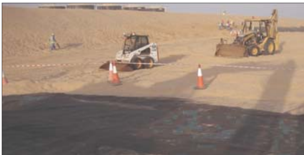
Area cleared of sand backfill, damaged Geocomposite net replaced, geocomposite liner inspected and tested for leaks
