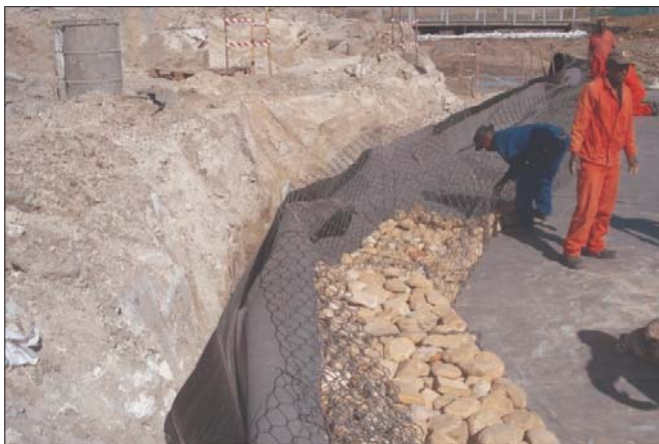
Hand filling of gabions
