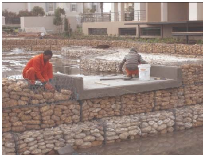
Installation of weirs between each pond
